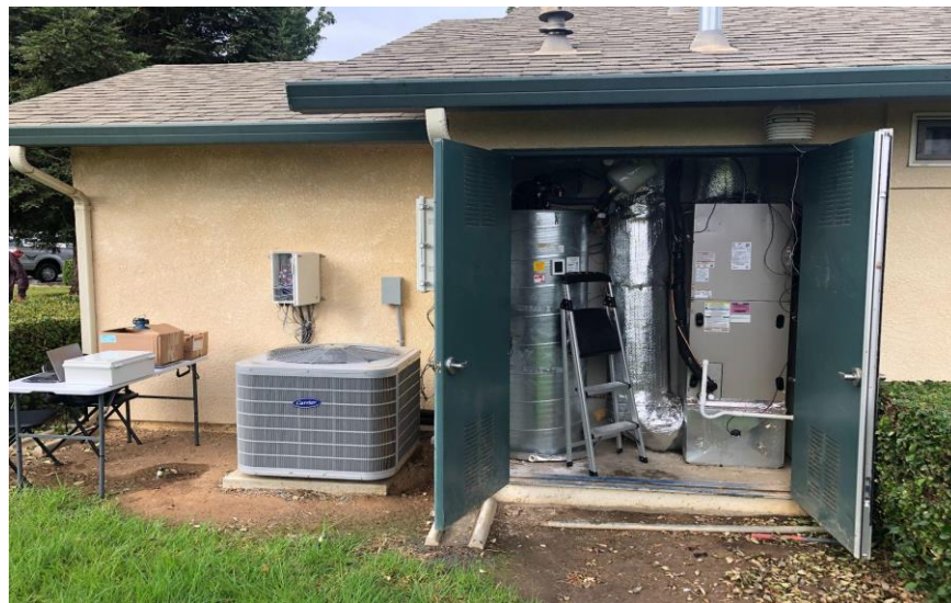
Figure 5. Completed MFHP system installation with all three components
